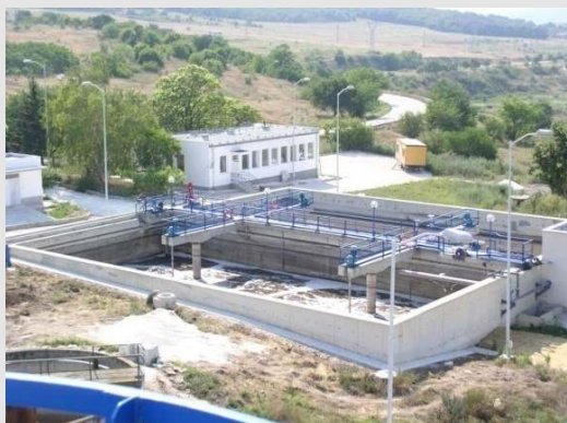
Biogest-wastewater treatment plant of the Bulgarian town Beloslav (20,000 p.e.).
