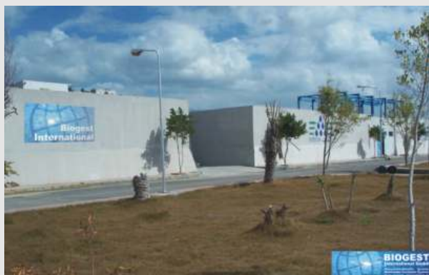
Biogest-wastewater treatment plant of the Egyptian village „Amreya“ located next to Alexandria. The hydraulic load is approx. 5,000 - 6,000 m 3 /d, being treated by totally three (3) SB-Reactors. Aeration and mixing is performed by floating BSK ® -Turbines Ø 2.50 m.
