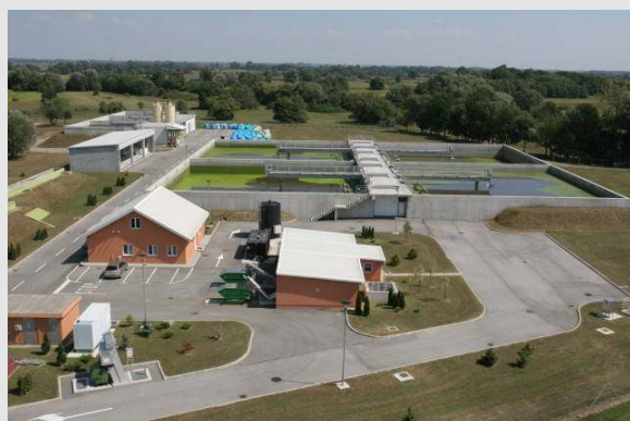
Bird-eyes view of the wastewater treatment plant being designed and realized by Biogest International GmbH for the Croatian town Koprivnica (100,000 p.e.) – operating according to the SBR-process (4 reactors).
