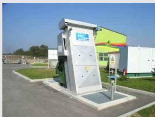
Automatic coarse screen for mechanical pretreatment of wastewater. Completely made of stainless steel in order to guarantee a long-life, no corrosion and proper operation.
