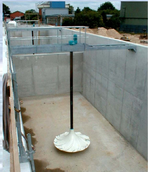
Picture no. 9: HyperClassic®-Aerators for a SB-reactor. Totally four reactors are combined to a wastewater treatment plant (65,000 p.e.).
