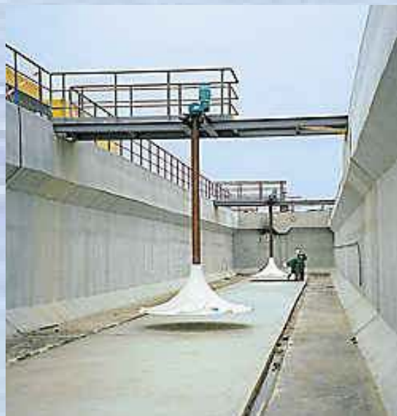
Picture no. 3: HyperClassic®-stirrers in a denitrification tank.
