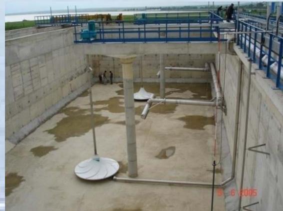
Picture no. 9: HyperClassic®-Aerators for a SB-reactor. Totally four reactors are combined to a wastewater treatment plant (65,000 p.e.).
