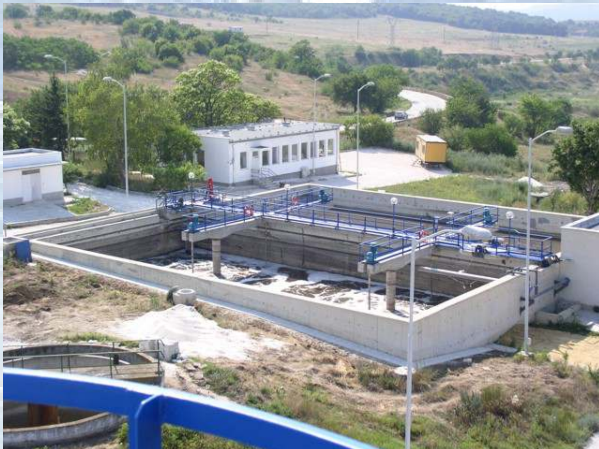
Picture no. 1: HyperClassic ® -Aerators for a SBR-wastewater treatment plant (25,000 p.e.)
