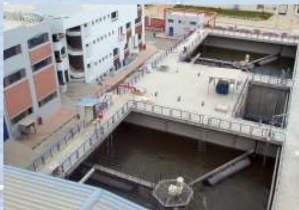
Photo no. 3: Typical example for the application of floating BSK-Turbines for industrial wastewater treatment. The so called "CMC-project" near Cairo (Egypt) is operating a 2-stage SBR designed and equipped by Biogest International GmbH.
