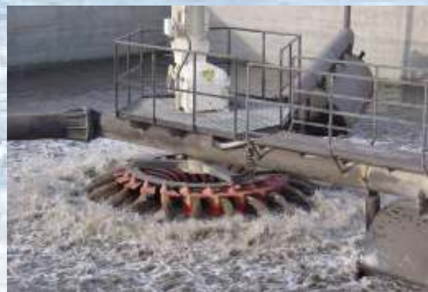
Photo No. 2: The BSK-Surface Aerator is the standard equipment for the OTR-plants. Totally six sizes (900-3,150 mm) are available for a wide range of OTR-sizes.
