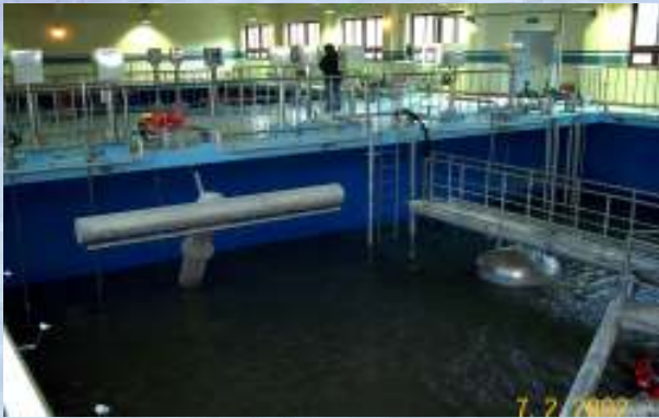
Photo no. 4: Two-stage OTR-treatment system for the Korean town "Muju". Design and equipment were performed by Biogest International GmbH. Connection load is 15,000 p.e.
