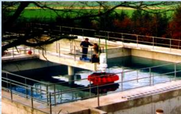
Photo No. 1: BSK-Surface Aerator for a tannery in Germany (two SBR-stages are operating in change). The high efficient oxygen input needs not only the requirements of the extremely polluted wastewater, but guarantees a sufficient oxygen supply - even under peak load conditions.
