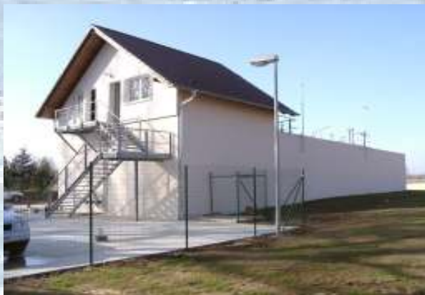
Photo no. 6: Two-stage OTR-treatment system for a village with industry in Saxony (Germany). Connection load is 2,400 p.e.
