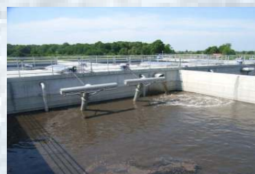
BSK®-Decanters for the Croatian-WWTP Koprivnica
