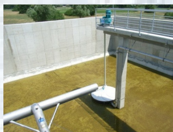
BSK®-decanter operating in a wastewater treatment plant next to Basel (Switzerland)
