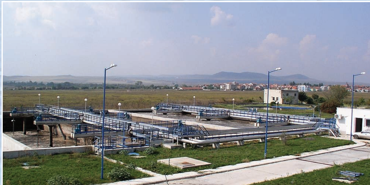
View of the 4-street SBR-WWTP of the resort SUNNY BEACH
