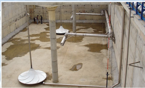
SB-reactor during assembly phase (mixers and decanters)
