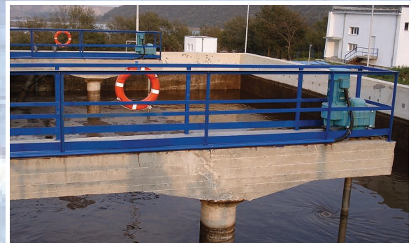
Service platform with drives for HyperClassic-stirrers
