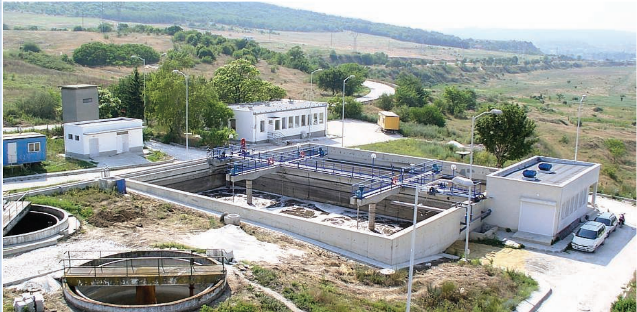
View of the 2-street SBR-WWTP of village BELOSLAV
