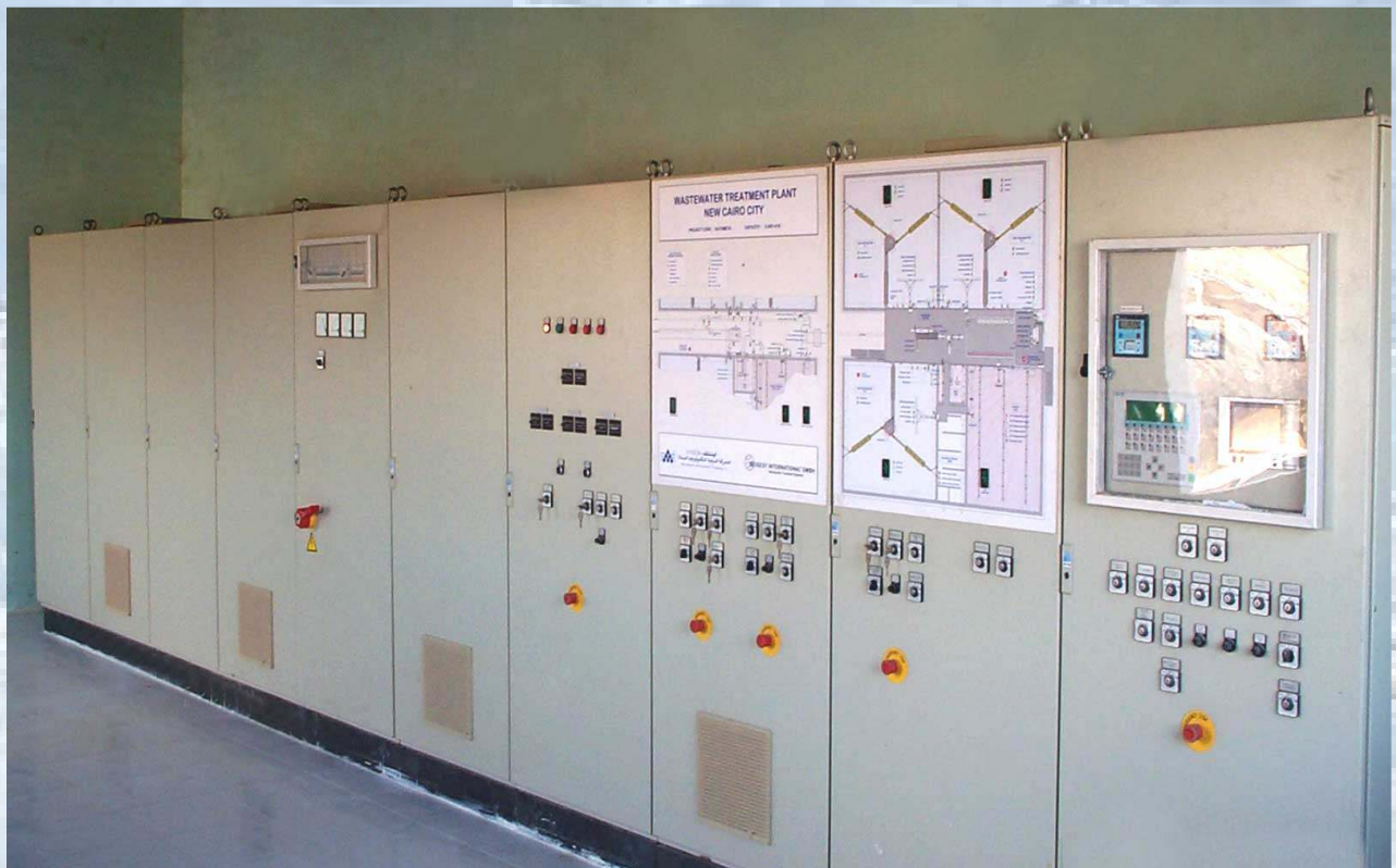
Central control paddle for automatic operation including remote control from the Cairo-service station
