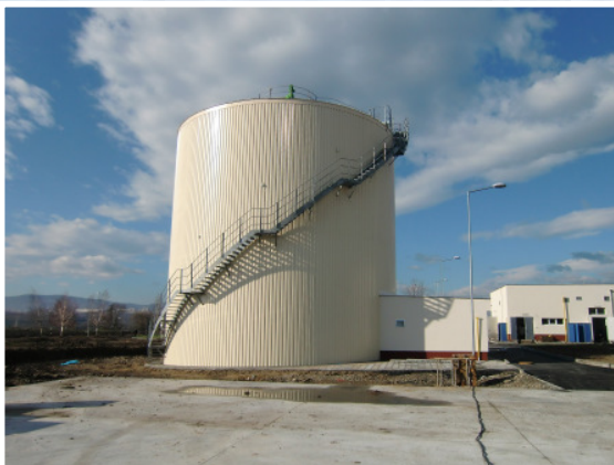
Sludge digester for anaerobic treatment of biological excess sludge and primary sludge for production of methane gas
