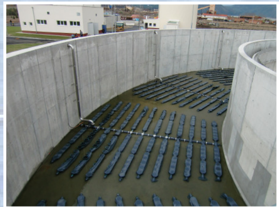
Installation of fine bubble disc aerators (including protection covering before start-up)
