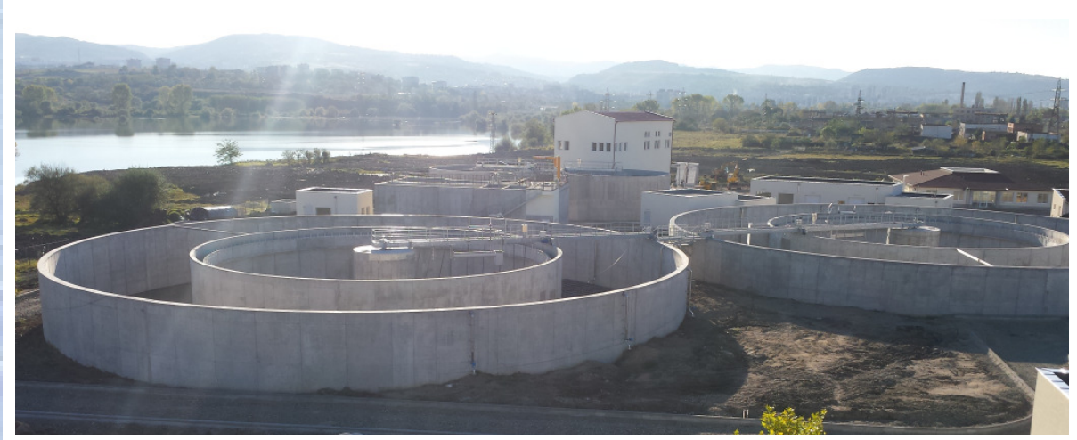
Wastewater treatment plant of town Kardzhali just before start-up
