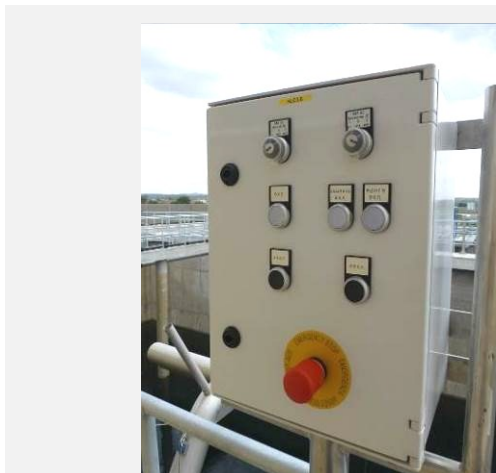
Example of a local switchbox for one BSK®-decanter. The cabinet could be produced by use of glass fiber reinforced plastic (GRP) or stainless steel. Moreover, the front side could be covered by a moveable door with glass-window (for protection of dust).
