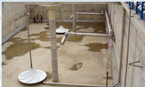
SB-reactor during assembly phase (mixers and decanters)
