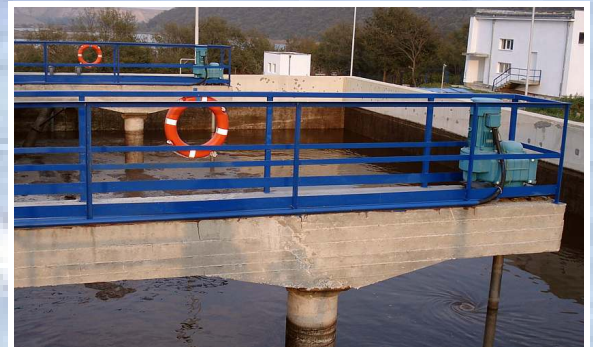
Service platform with drives for HyperClassic-stirrers
