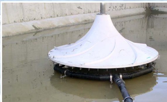
Mixer-body with aeration pipe
