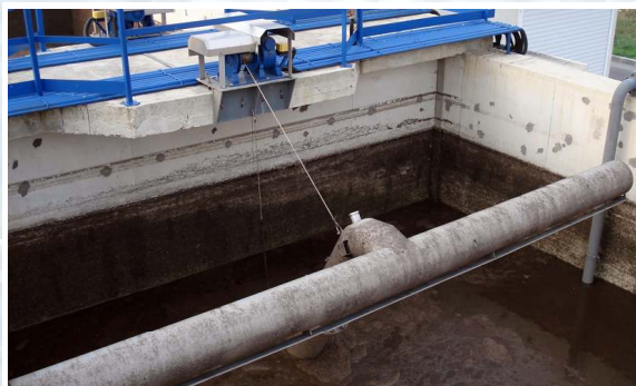
Clear water decanter with electrical winch
