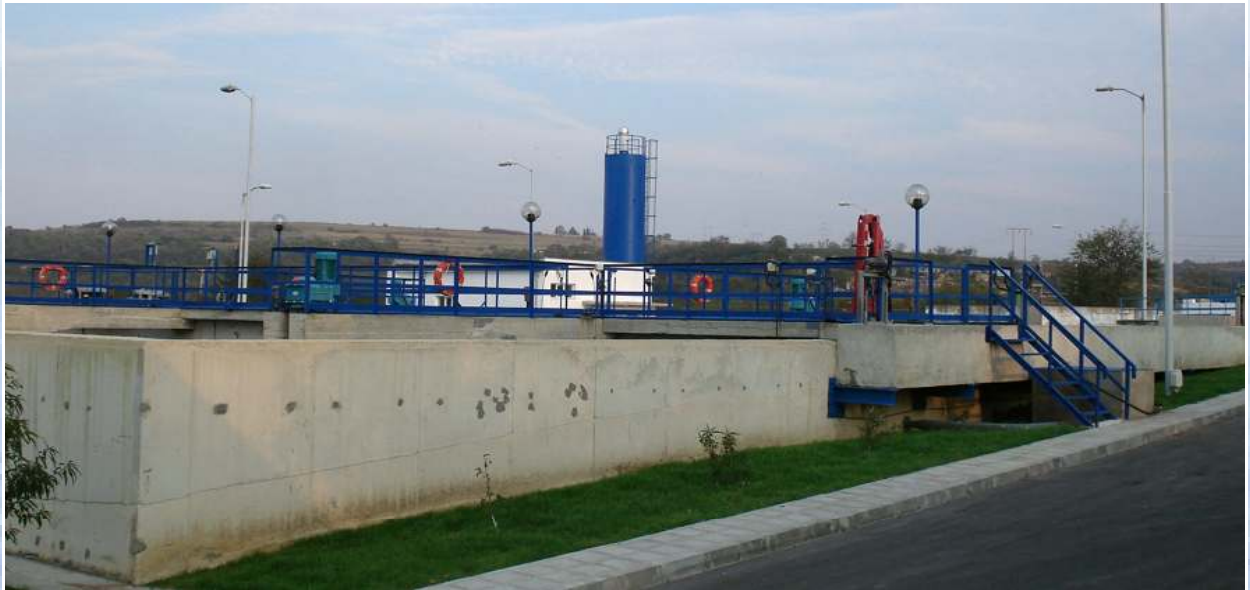
View from the access road to the two SB-reactors
