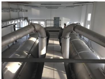
2-street compact pre-treatment station, completely made of stainless steel including high-performance "Walzensandfang"
