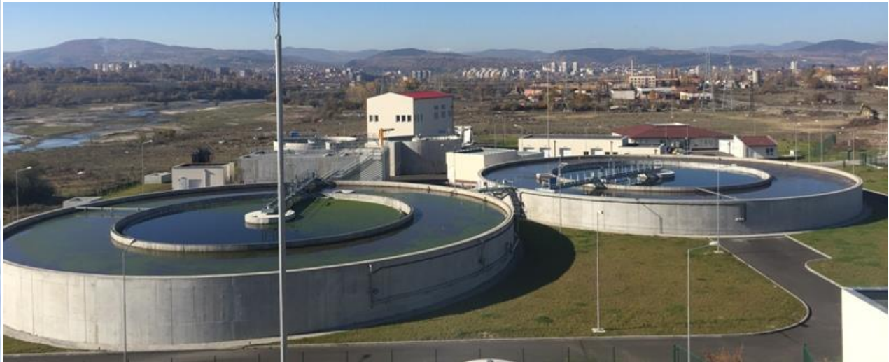
Biological wastewater treatment plant of town Kardzhali after start-up. Realized by Biogest International GmbH in cooperation with a local general contractor.
