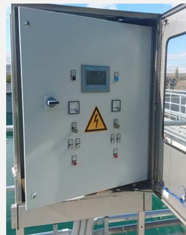
Example of a local stand-alone control system (plug and play), operating two (2) BSK®-decanters completely independent to the customer's PLC. This cabinet is equipped with a moveable cover with glass window. glass-window (for protection of dust).
