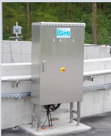
The control of a BSK-decanter can be performed by a local switchbox (on the left) or by an own control cabinet with PLC (middle and on the right)
